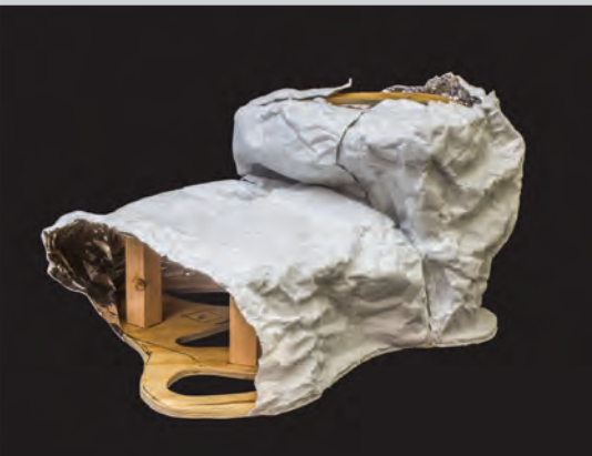
1 Form Contour Sheet around understructure.
